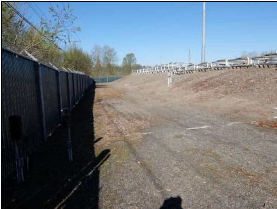
PHOTO TWO: WESTERLY VIEW OF ACQUISITION AREA
