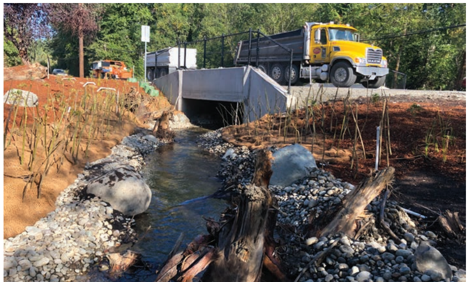
Ebright Creek Culverts Project, designed by OCI and constructed in 2021
