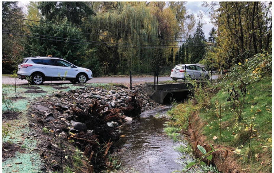
NE 192nd St Culvert, designed by OCI and constructed in 2018
