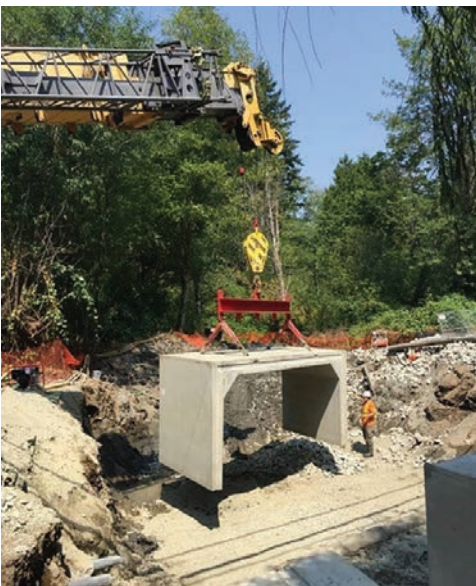
During 2018 construction of 192nd St Culvert
