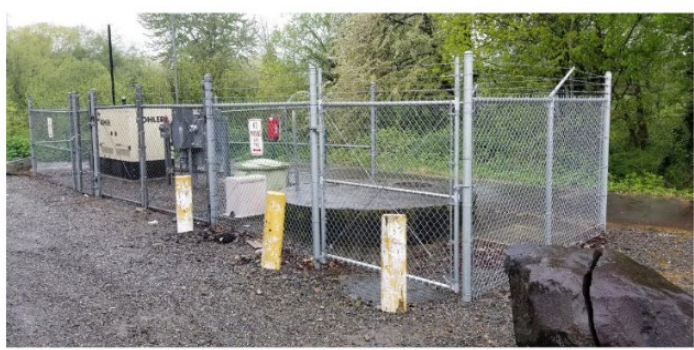
Lift Station 2 and 6 Panel Replacements
