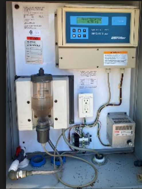
Chlorinator/Analyzers
