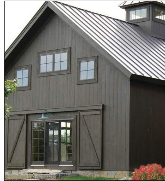
Standing Seam Roof
