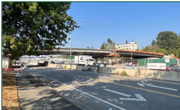
Main Street Bridge Demolition video:
