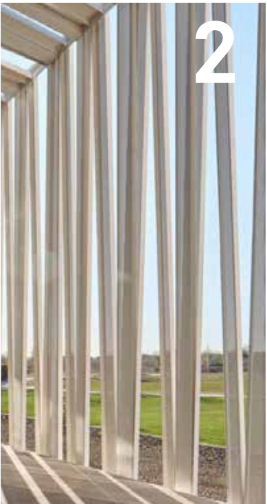
Metal panel facade system set off of the face of building to create depth and shadows
