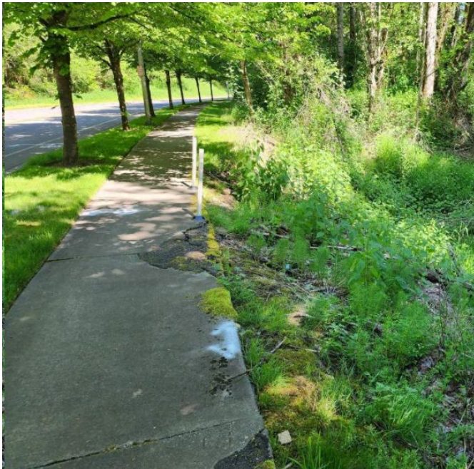
West Valley Highway Sidewalk Repair
