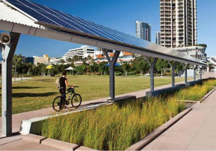
Solar panel roofs with rainwater collection
