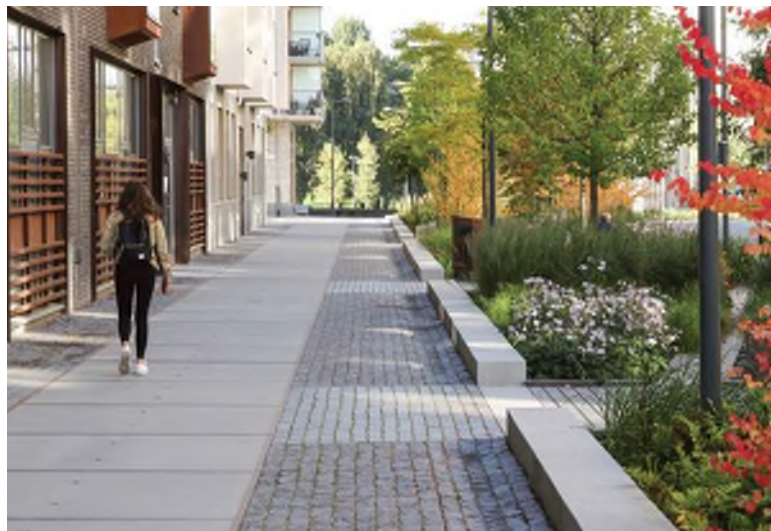
Sidewalk | Unit Pavers at Utility Corridor | Plantings provide pedestrian access and organization/access of utilities.
