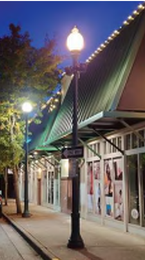
Existing Light Pole
