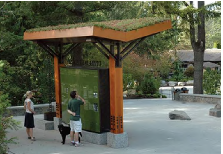
Green roofs on structures clean and collect rainwater
