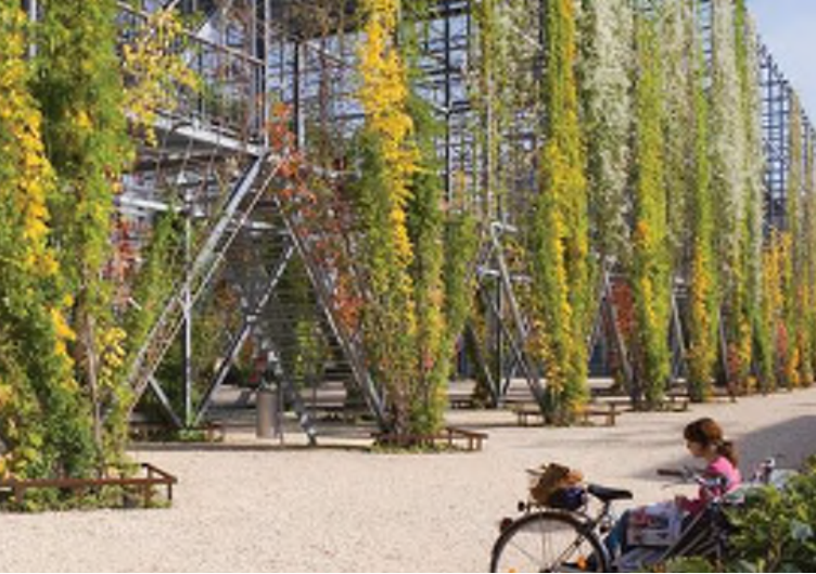
A hop trellis inspired shade/canopy structure provides flexible seating and beer garden opportunities beneath.
