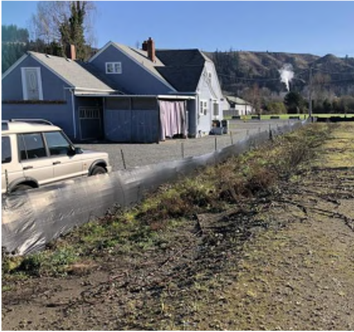
2 LOOKING EAST - FROM NE CORNER OF THE SITE
