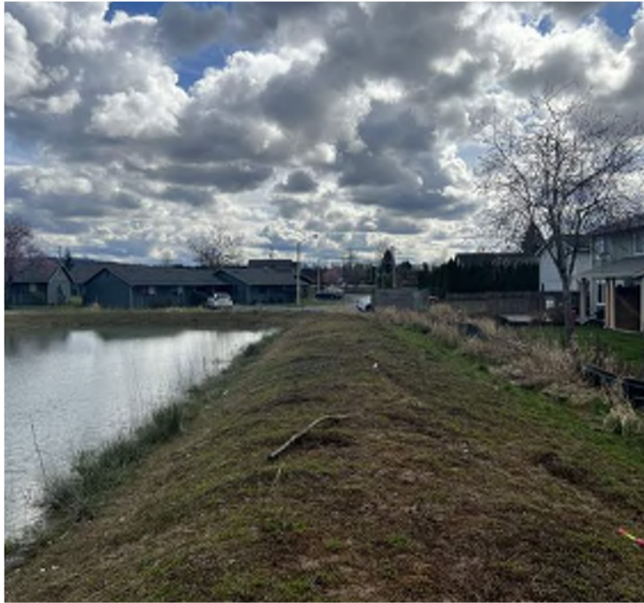
5 LOOKING SOUTH - FROM SW CORNER OF THE SITE
