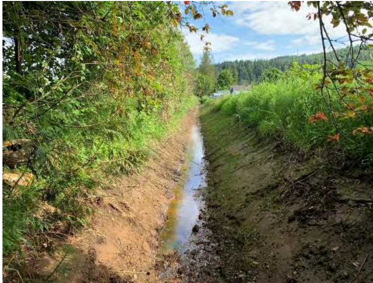
Picture 2. Ditch 1. Facing North Toward 60 th Street East. (Taken 6/1/20)
