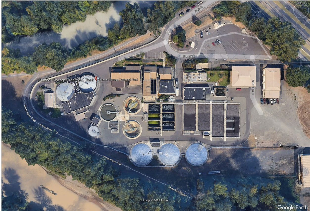
Figure 3-5: Wastewater Treatment Facility - 13114 63rd Street East
