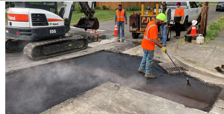
Pavement Patching Overlay
