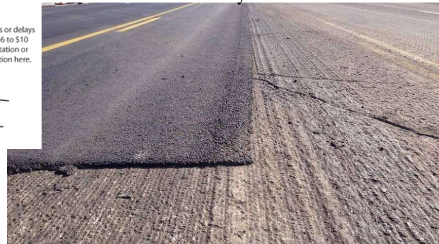
Pavement Patching Overlay
