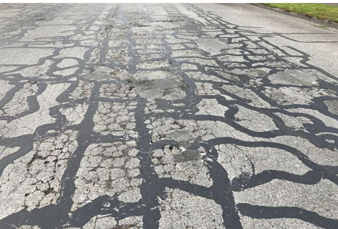
Crack Seal
