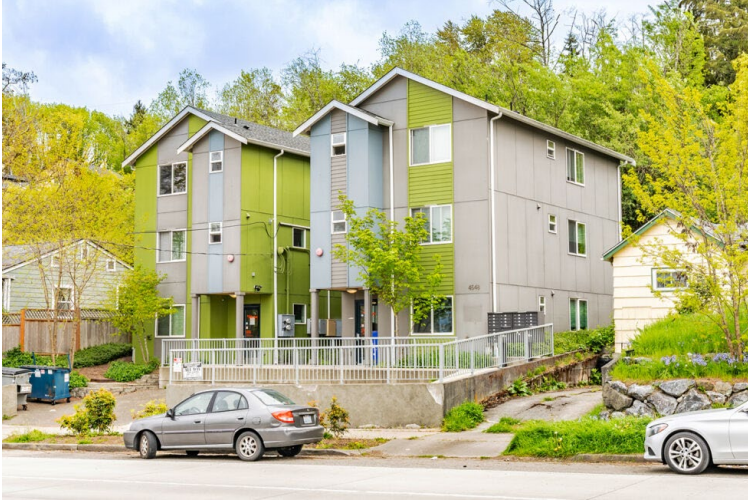
Westward Studios, a 17-unit co-living development in Seattle acquired and renovated by Great Expectations
