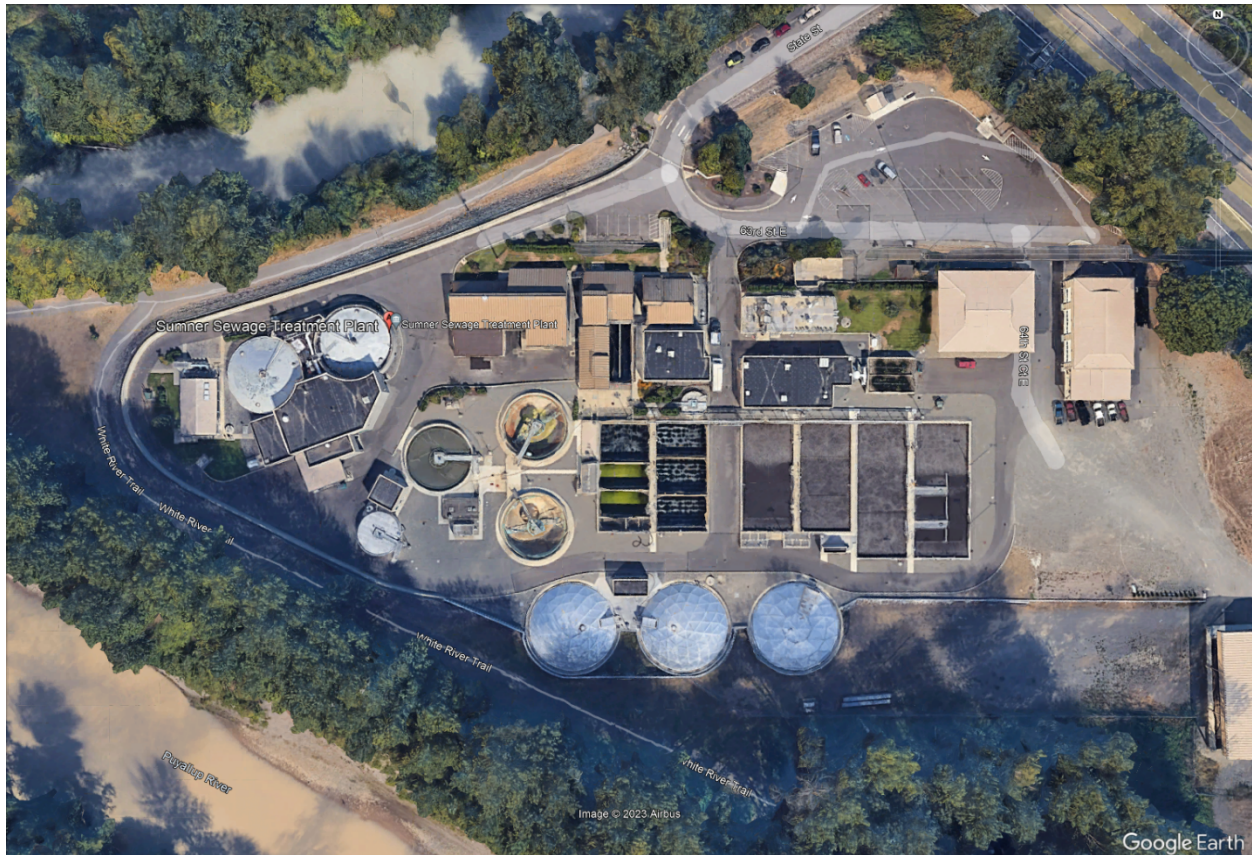
Figure 3-5: Wastewater Treatment Facility – 13114 63rd Street East
