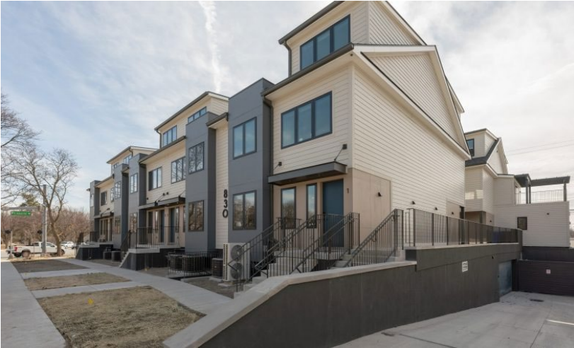
Prentice 4M, a developer of work-live Townhome buildings, announced the opening of the its first 4M campus in Ann Arbor. Offers a 7,500-square-foot space called The Flex in the center of the building, an open space for networking, social activities, exercise and fitness classes, and pop-up events.
