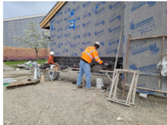
Mountain View Middle Construction
