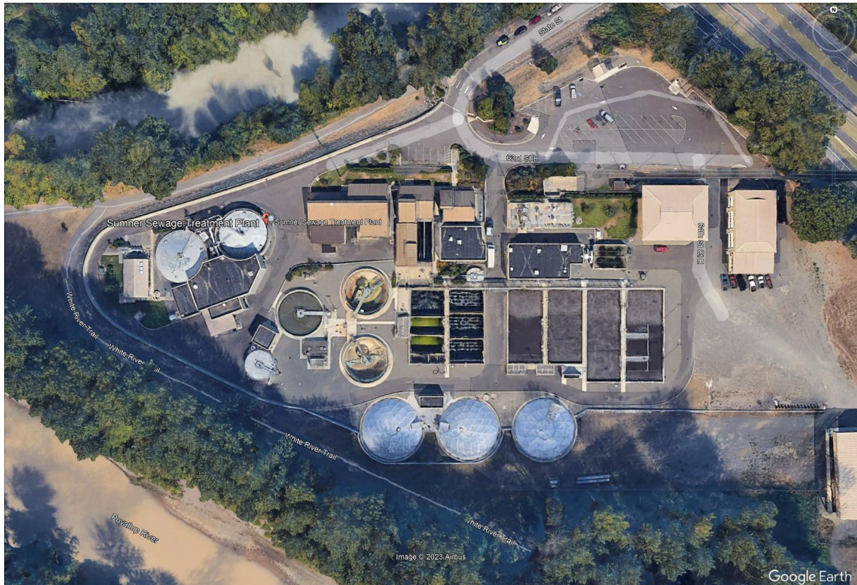
Figure 3-5: Wastewater Treatment Facility - 13114 63rd Street East
