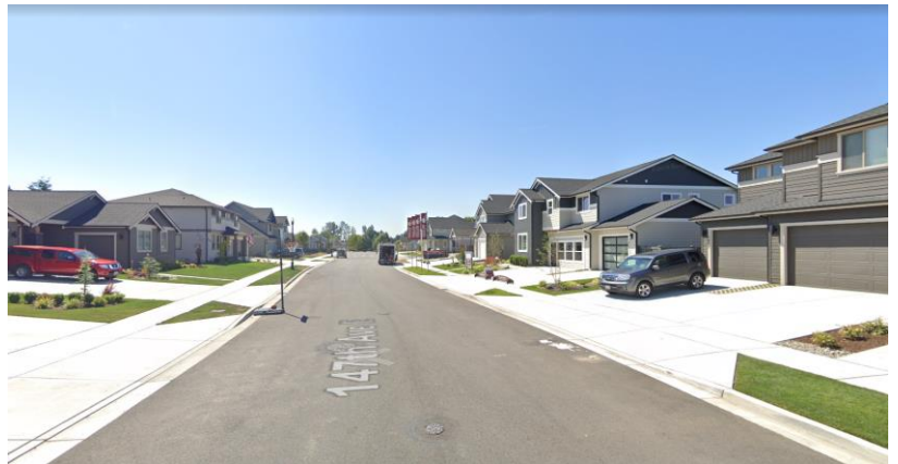
Existing 147th Ave E Improved to City Street Standards (from Google Street view)
