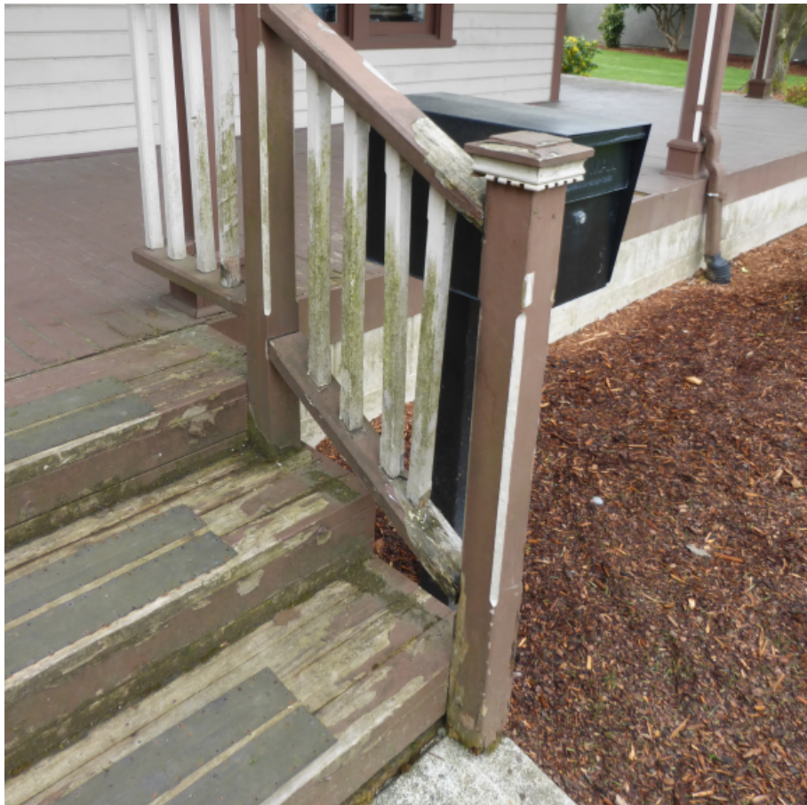
Example of deteriorated wood at porch stairs and railings to be replaced.
