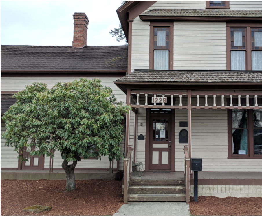
Existing non-accessible porch and front door
