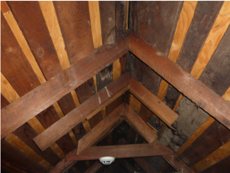
Existing attic space
