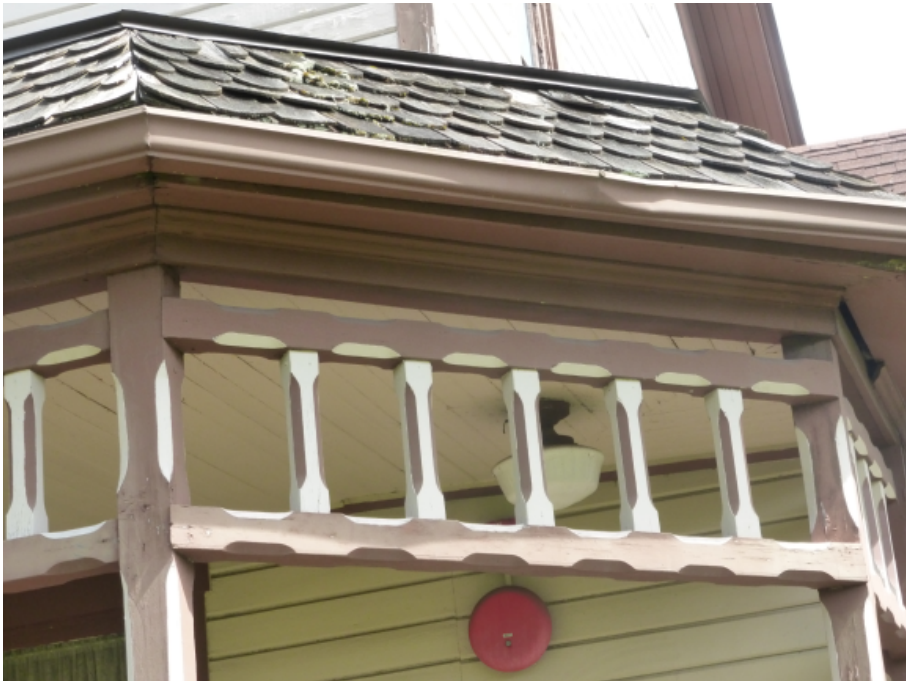
Character defining features: Wrap-around veranda, roof, and wood millwork
