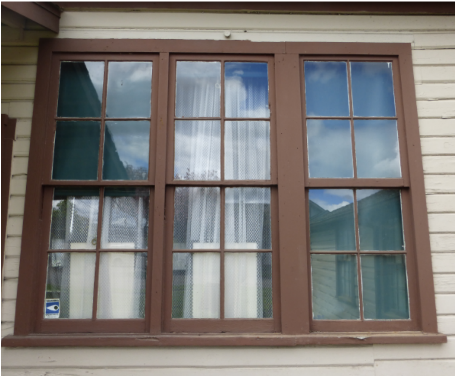
Character defining features: Historic wood double-hung windows and lap siding
