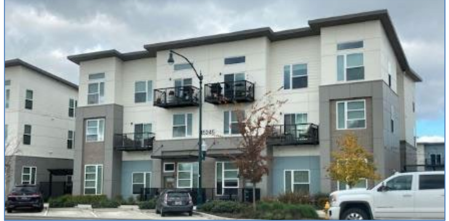
The Main + Lofts – East Main, Sumner: 3 story = 32 du/ac
