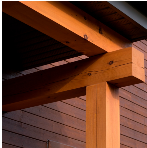
7 Wood Beams, Posts & Roof Corbels
